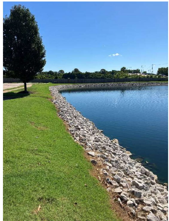
Right: Rip rap on the banks of a retention basin extends below normal water level >
